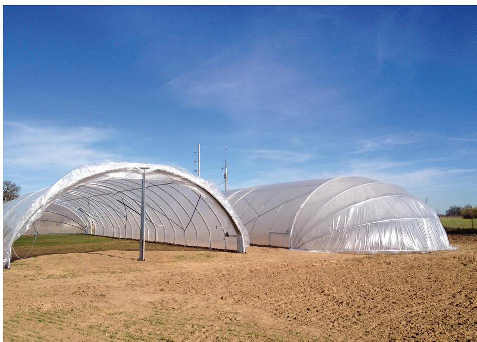
eliminate the need to back up while positioning the equipment inside the structure. Leon responded by designing a detachable end wall that mates with the end hoop. This end wall uses four bolts to secure it to the structure. While effective, this particular detachable design requires two or more people to remove and reattach the end wall with each use of equipment.
