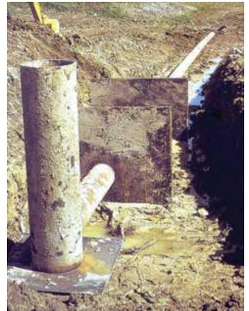
Fig. 3. A drop inlet spillway with anti-seep collars (USDA-NRCS Agriculture Handbook 590 "Ponds – Planning, Design, Construction").
